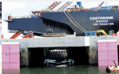
Wheel fenders are widely used on exposed corners to help ships maneuver into berths and narrow channels such as locks and dry-dock entrances.
