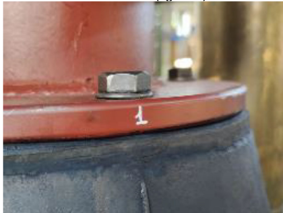
Figure 8: Visual inspection test b (100K Cycles @ 35% compressions) (Politecnico Milano)
