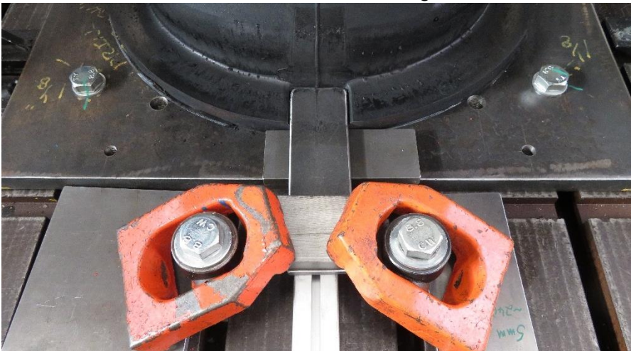
Photo 3- Clamp to replace the bolt
